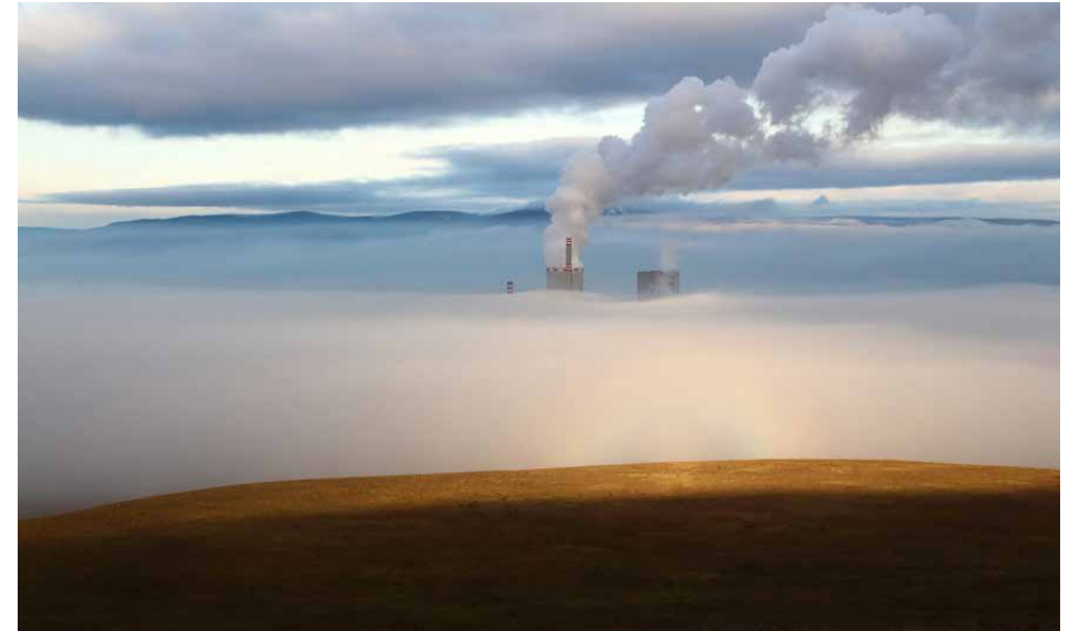
Photo 2.17 One of the large brown coal thermal power plants in Ledvice, owned by the energy company ČEZ, is situated in the Podkrušnohorská Basin, where brown coal is mined. As it is a valley surrounded by mountains on both sides, frequent inversions occur here from autumn to spring, trapping pollution closer to the ground. However, the power plant chimney and cooling towers peek above the inversion cloudiness in this photograph. Brown coal power plants, besides emitting sulfur dioxide, carbon dioxide, and dust, are also significant sources of heavy metals, including arsenic, which then accumulate in the residues from flue gas cleaning (Petrlík 2010). Photo: Daniela Endrštová
