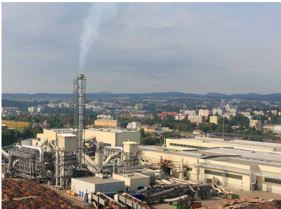
Photo 4.4: Kronospan Jihlava, a manufacturer of chipboards, was the largest polluter with cancer-causing chemicals according to data published in IRZ (Czech PRTR system) for several years, e.g., for the reporting year 2009 (Petrlik 2013).
