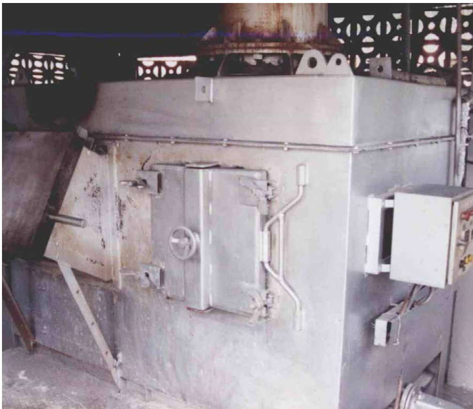
Photos 4.36 – 4.37: Small medical waste incinerators built in Asia are not very different from those in Africa. In the photos taken in 2005, there are two such waste incinerators in Pakistan, Peshawar and Islamabad (Khwaja and Petrlik 2006). Photo: Jindřich Petrlik, Arnika
