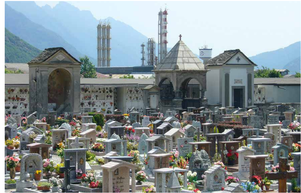
Photos 3.1 and 3.2: Chlor-alkali plant in Pieve Vergonte, Italy was found to be a large source of mercury (Fantozzi et al. 2021)* PRTR can clearly demonstrate to public large sources of mercury, and Mercury Toolkit (UNEP Chemicals 2013) is an important tool developed within framework of the Minamata Convention to support reporting into PRTRs about mercury releases and transfers in wastes. Photo: Legambiente, 2006
